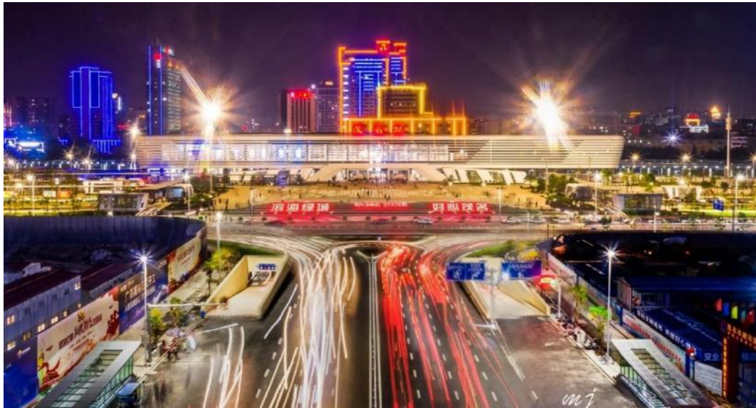
Fig.10: Example of Roads
