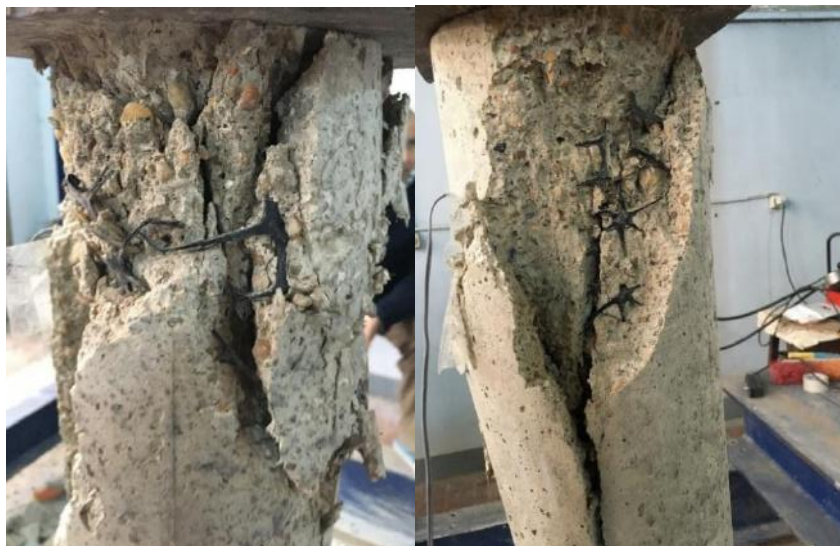
Fig.8: Failure of Carbon fibre concrete piles with geogrid confinement
