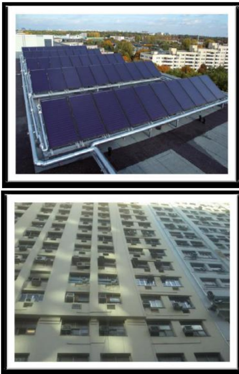
Fig.2. Thermal Solar Array and Split Coolers with Compressor Operation.
