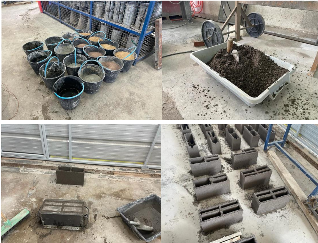
Fig.2 – (a) Separation of materials, (b) Finished mass for block molding, (c) Manual mold for block molding, (d) Molding of the concrete blocks.
