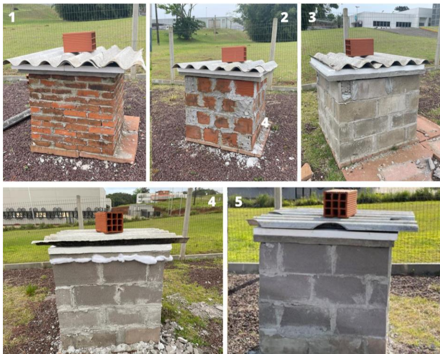
Fig.5 – Building of the prototypes completed.
