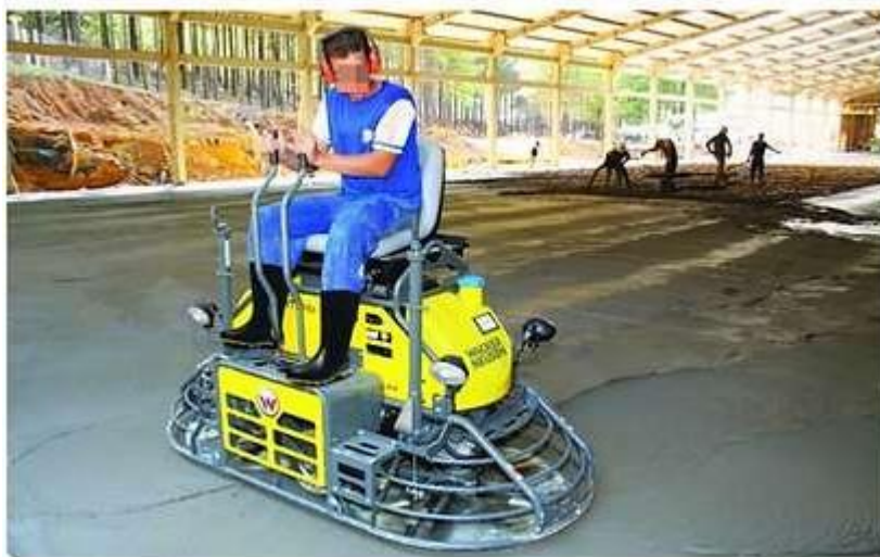
Fig.3 – Floor leveler used in construction. Source: ERGOTRIADE (2021)
