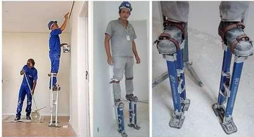
Fig.2 – Mechanical legs used in civil construction. Source: ERGOTRIADE (2021)
