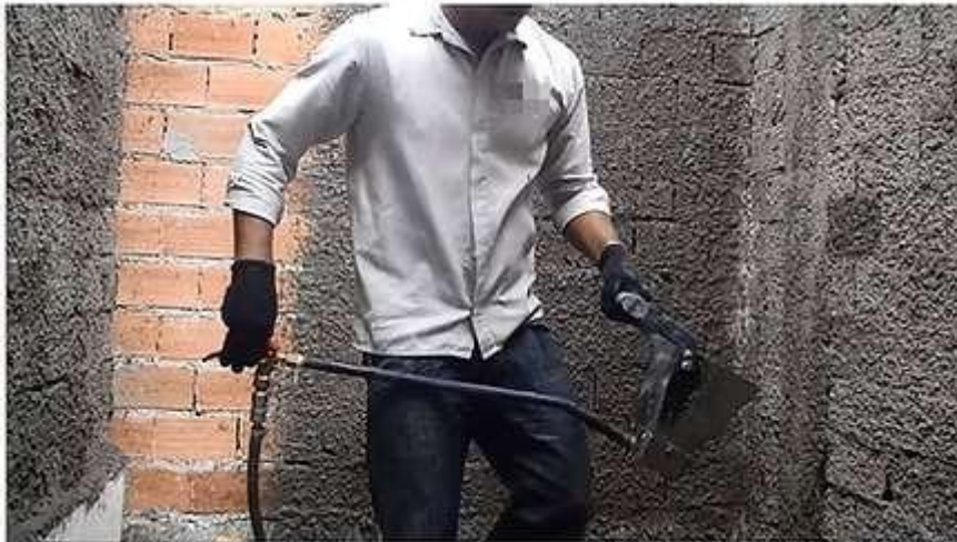
Fig.4 – Plastering and plastering machine used in construction. Source: ERGOTRIADE (2021)
